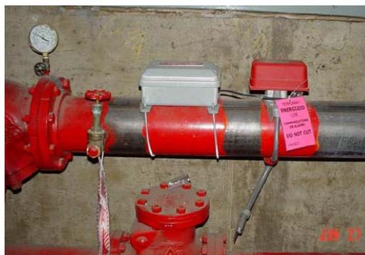
**Figure 6-15. A wireless transmitter installed at Rocky Flats.**
