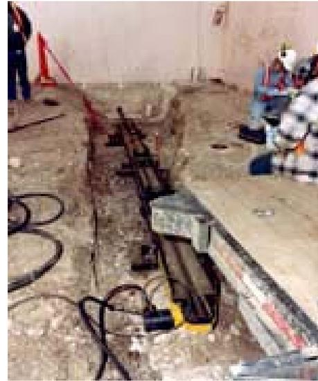
**Figure 6-1. Environmental sampling using HDD at Building 865 at Rocky Flats.**
