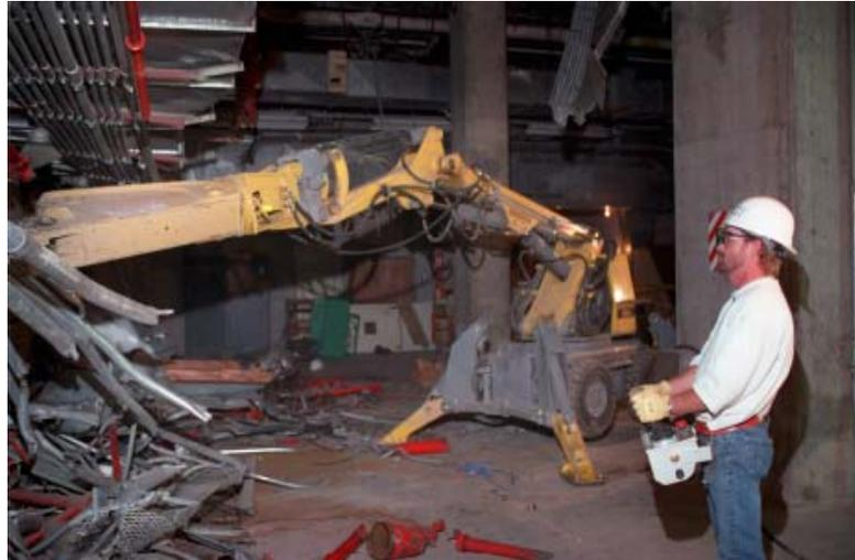
**Figure 6-8. The Brokk 250 performing demolition at INEEL.**
