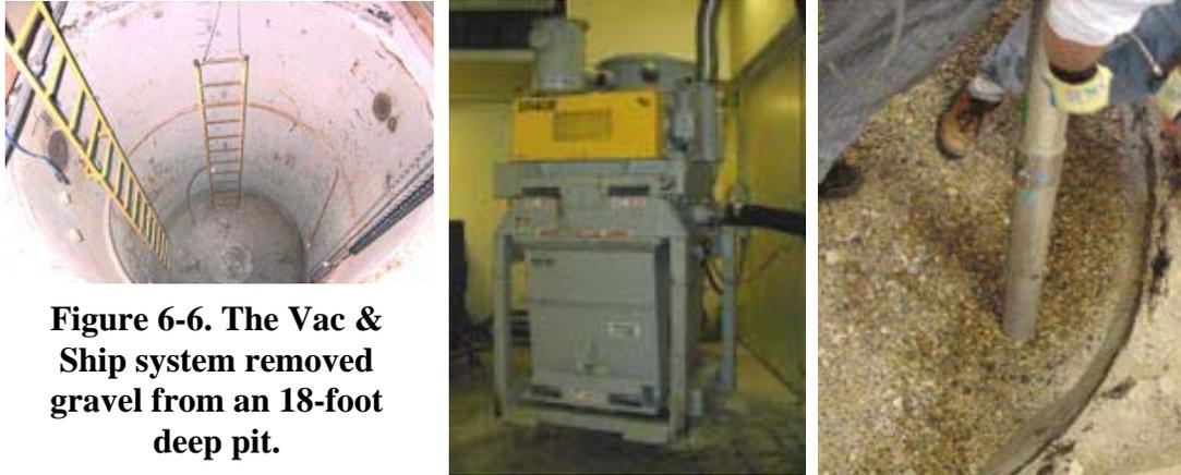
**Figure 6-6. The Vac & Ship system removed gravel from an 18-foot deep pit.**
