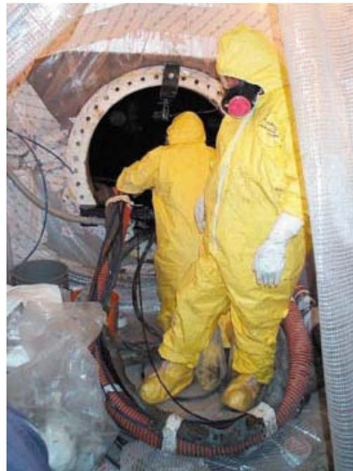
**Figure 6-7. Workers introduce the remote-controlled track vehicle to remove sludge from a waste tank at Rocky Flats.**
