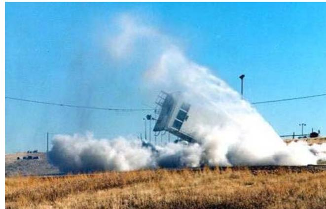
**Figure 6-10. Explosive demolition of a guard tower at Rocky Flats.**
