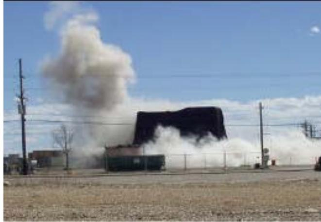
**Figure 6-9. Building 886 at Rocky Flats is shown draped in engineering fabric at the moment of detonation.**
