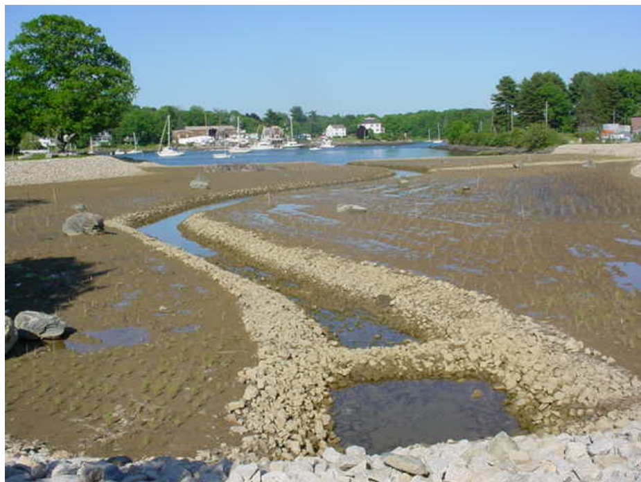
Salt Marsh Establishment After Consolidation and Backfilling
