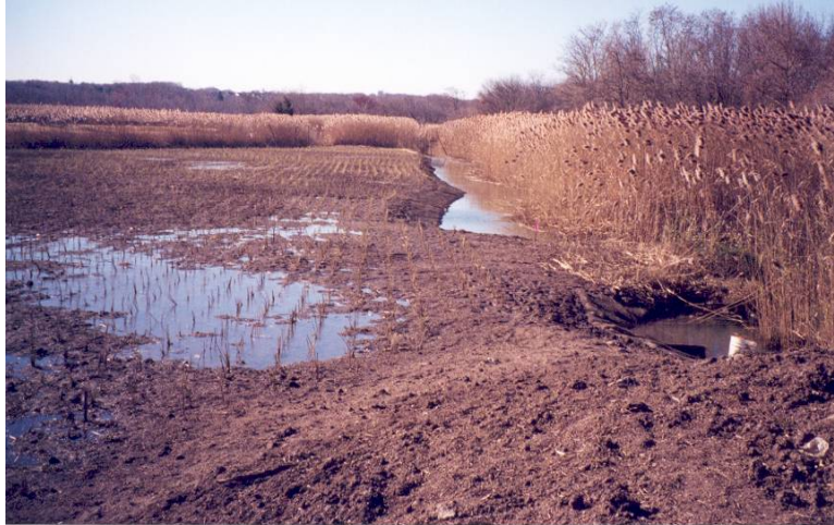
Figure 6-1. Site planting (courtesy of Charles Harman, AMEC Earth and Environmental).
