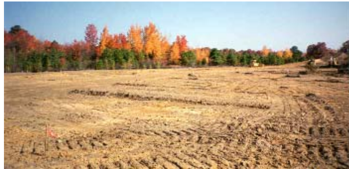
Figure 5-2. Process of developing the grade on a site and (background) example of the equipment used for grading (courtesy Charles Harman, AMEC Earth & Environmental, Inc.).
