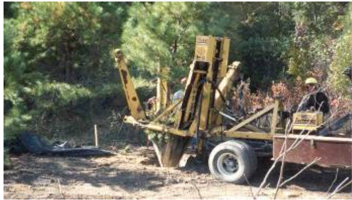
Figure 5-1. Planting equipment (courtesy Charles Harman, AMEC Earth & Environmental, Inc.).
