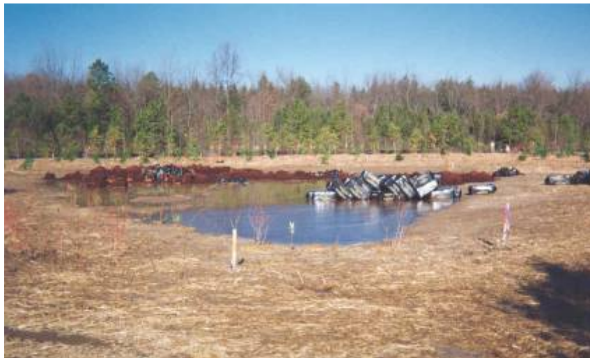
Figure 1-2. Wetlands creation in progress (courtesy Charles Harman, AMEC Earth & Environmental).
