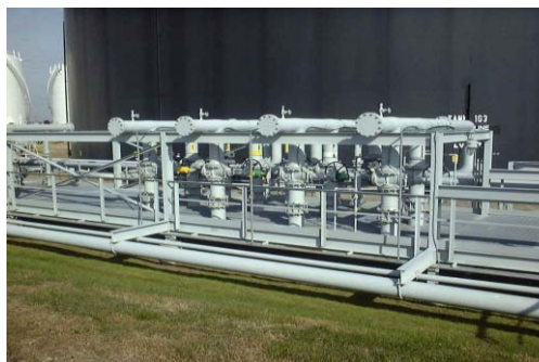
Distribution Piping and Manifold
