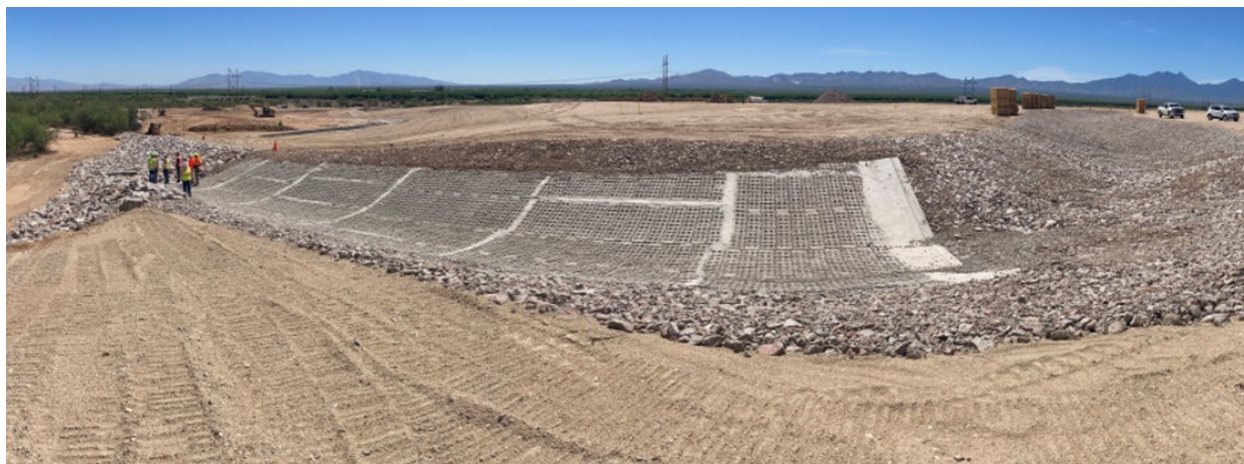
Figure 6-1. Articulated concrete-block-lined drainage channel installed as erosion control for the engineered cap.
