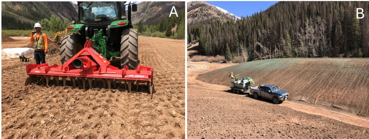
Figure 6-5. Kittimac tailings revegetation (A) and reseeded monofill (B).
