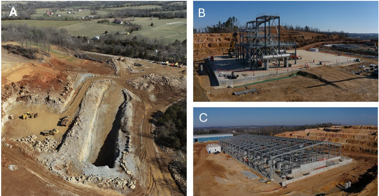
Figure 6-14. Construction of the new decline access (A), hydrometallurgical crystallizer facility (B), and Hydrometallurgical solvent extraction facility (C).
