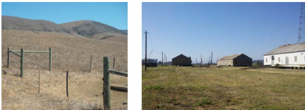
Figure 3-4. Negative effect of structures and utilities on EMI sensing for munitions.
