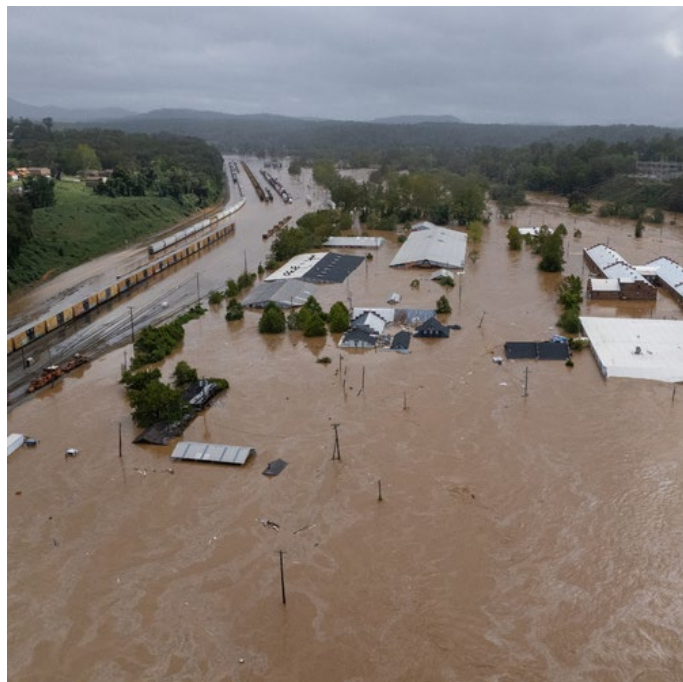
Figure 1-2. Aerial photo of floodwater inundating the Asheville River Arts District along Foundy Street on September 27, 2024.
