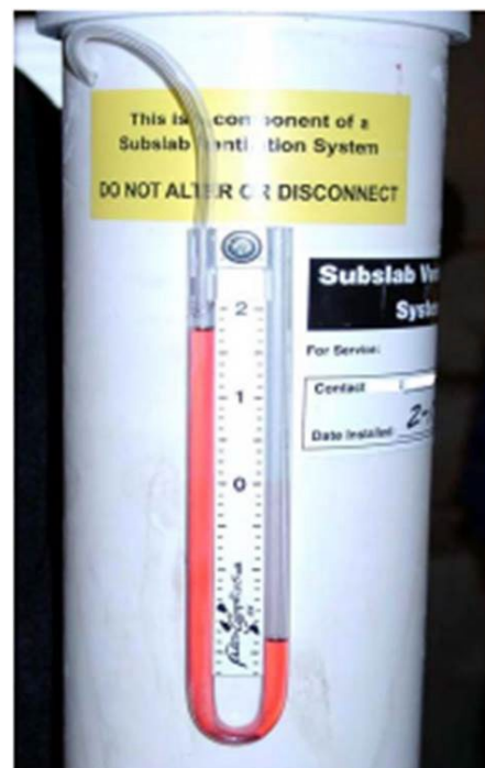
Figure 5. Typical U- tube manometer.
