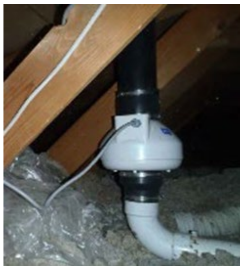
Figure 4. Blower installation inside attic, outside occupiable building envelope.
