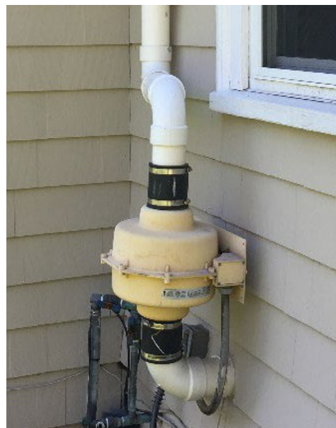
Figure 3. Blower installation outside building.
