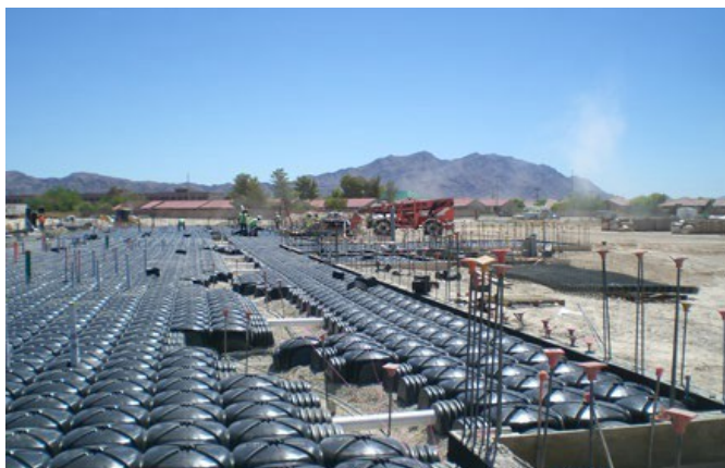
Figure 1. Aerated floor void space system.
