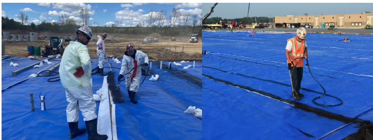
Figure 1. Application of asphalt latex membrane within the single-seam membrane seam (left) and single-seam membrane passive barrier with asphalt latex membrane over the top of the seam overlap (right).
