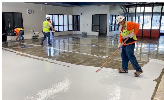
Figure 1. Application of epoxy floor coating to the prepared surface of an existing interior concrete slab.
