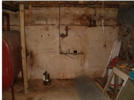
Commercial building basement, two AGI Universal Samplers Suspended, Summa can on floor; heating oil tank and workbench
