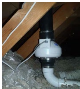
Figure 4. Blower installation inside attic, outside occupiable building envelope. Source: Clean Vapor, LLC
