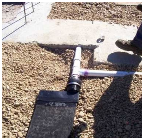
Figure 3. Photograph of a low-profile vent and vent pipes. Source: CETCO
