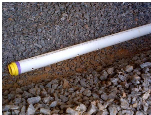
Figure 4. Photograph of mitigation system piping. Source: A. Rodak, Duncklee & Dunham, used with permission.
